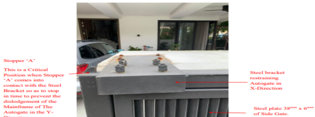
Photo 30 Side Elevation of Steel Bracket
